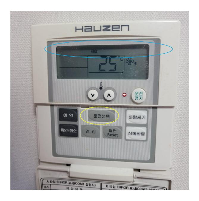
Here It says, "제습." This word means "Humidity Control." Clearly not very good at keeping the room cool. It, however, is useful for controlling the humidity on rainy days.
