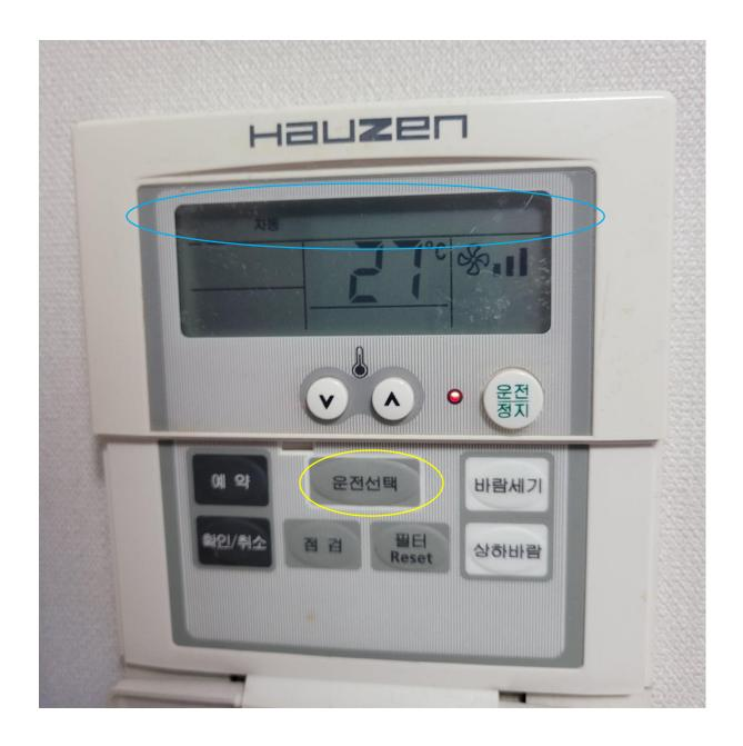
The word in the top row this time is "자동." It means, "automatic." From my experience, it seems to automatically adjust the temperature to what the unit feels to be optimal.
