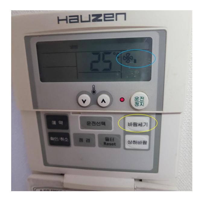
Next is fan speed. The button inside the yellow circle this time is called, "바람세기." It means "fan speed." The current picture does not have the capability to fully express the phenomenon that is happening here. What happens when you press that button when the box with the fan logo has three bars is that the bars cycle going one > two > three. I honestly am not familiar with what that does.
