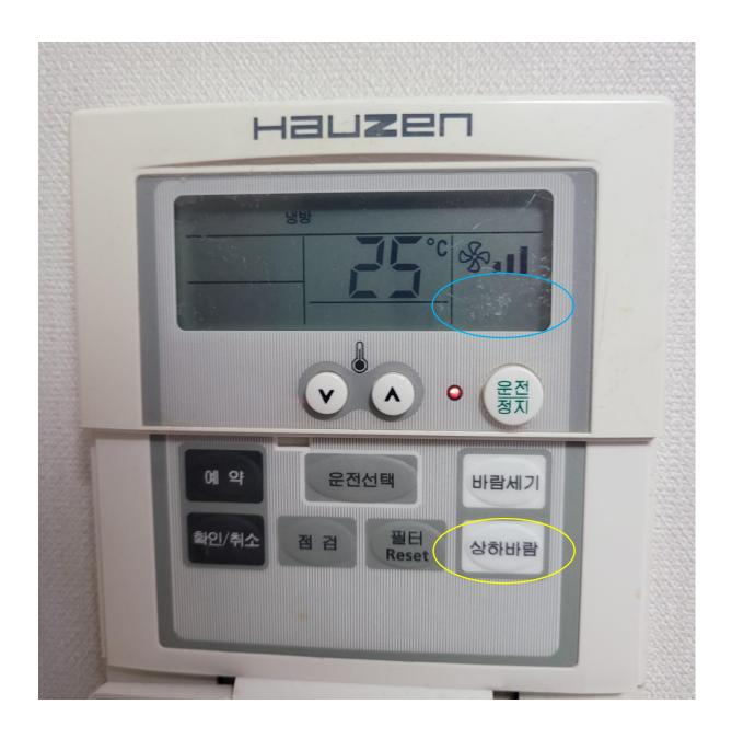
Last thing. We have "상하바람." This controls the vertical axis of the air conditioner. You can set it to move and then stop it when it faces what you personally deem to be most optimal. A mark will appear in the encircled area.
