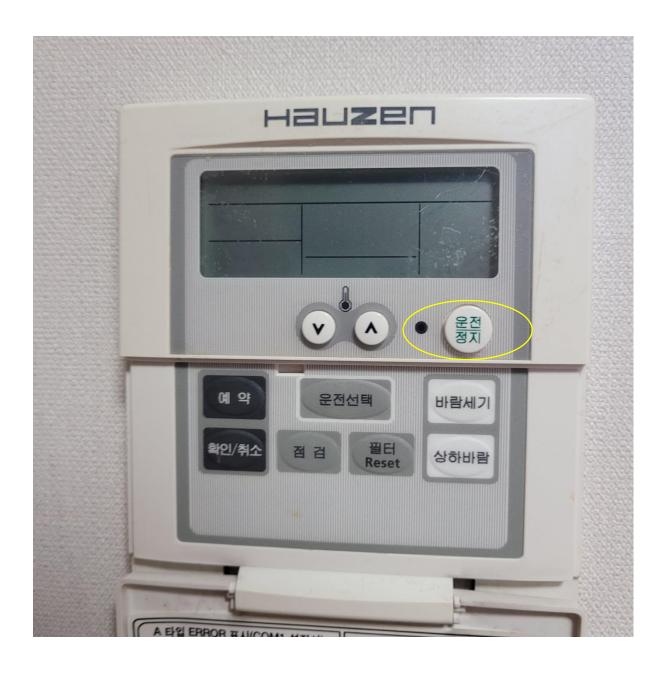
This is what the Air-con unit controller looks like when it is off. When you press the encircled button (it says On/Off) it turns on.
